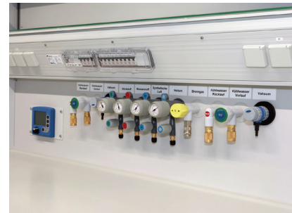
Controller installation within the media column
